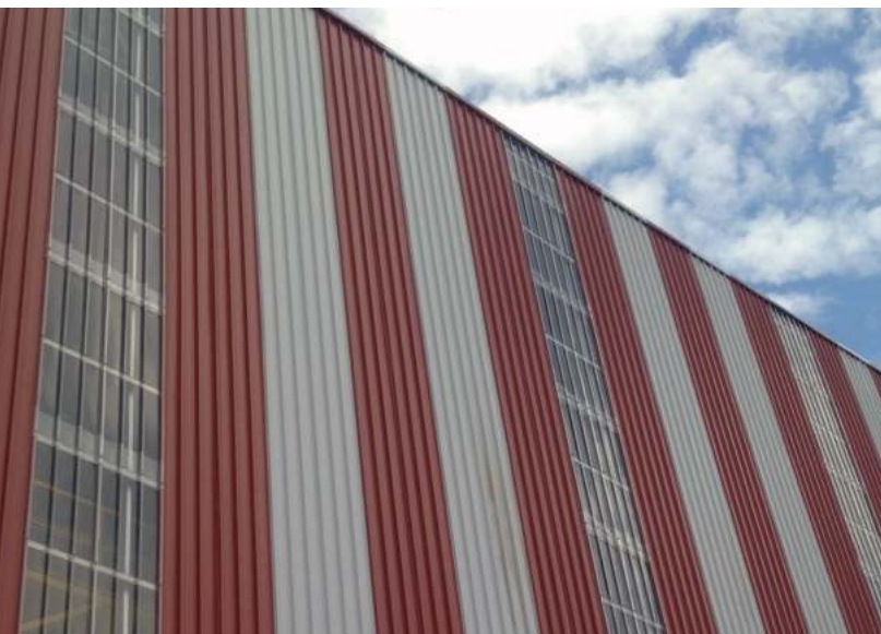
Southern Steel Seberang Prai
