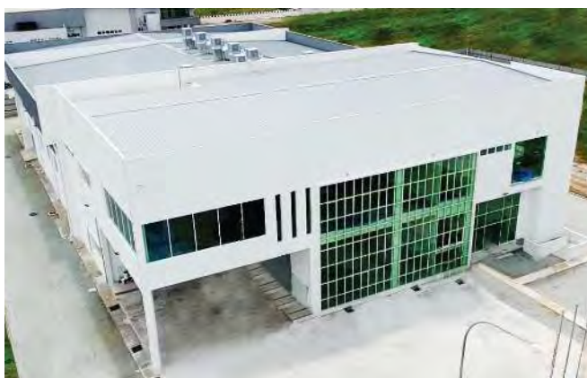
STREETS FOOD PRODUCTS SDN. BHD. Realcolor Primero 0.47mm TCT Superior Rib PU Metal 25mm in Pearl Grey
