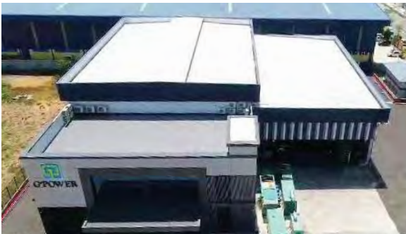
G POWER GENERATION SDN. BHD. Zincalume AZ150 0.53mm TCT High Rib PU Metal 25mm
