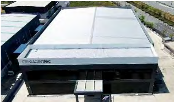
ASCENTEC ENGINEERING SDN. BHD. Aluzinc AZ150 0.47mm TCT High Rib PU Foam 25mm
