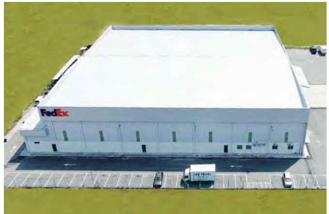
FedEx - FEDERAL EXPRESS SERVICES (M) SDN. BHD. Aluzinc AZ150 0.47mm TCT Clip Lock 672
