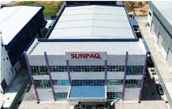
SUNPAQ SDN. BHD. Aluzinc AZ150 0.53mm TCT High Rib PU Aluminium 25mm
