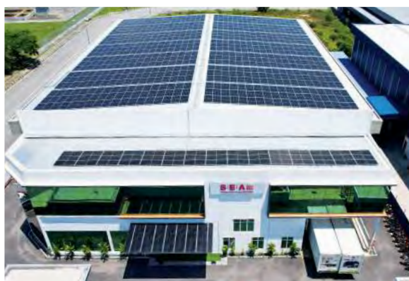
SEA ASIA PACIFIC SDN. BHD. Aluzinc AZ150 0.40mm TCT High Rib PU Metal 25mm
