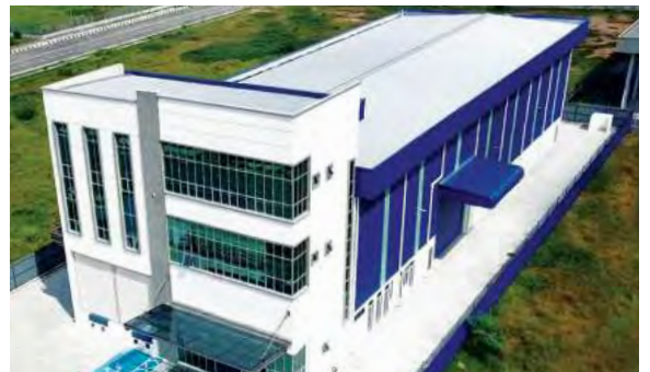
DSV SOLUTION SDN. BHD. Aluzinc AZ150 0.47mm TCT High Rib PU Aluminium 25mm
