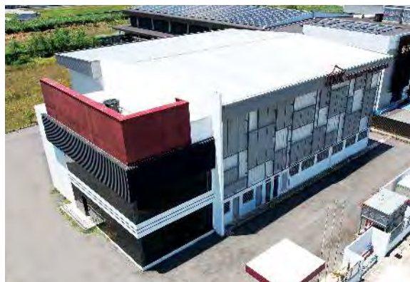
HNK ENGINEERING SDN. BHD. Aluzinc AZ150 0.47mm TCT Superior Rib PU Aluminium 20mm
